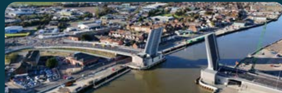
Herring Bridge Crossing
