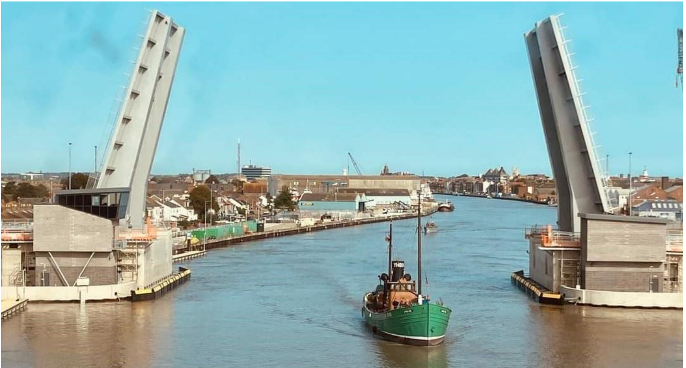
Herring Bridge viewed from S (seaward)
