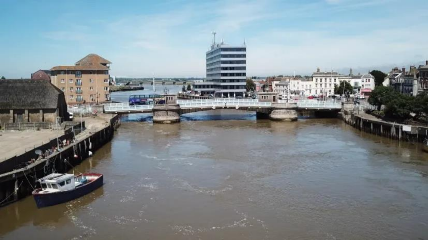
Haven Bridge viewed from SE (seaward)
