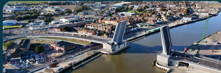
Herring Bridge Crossing
