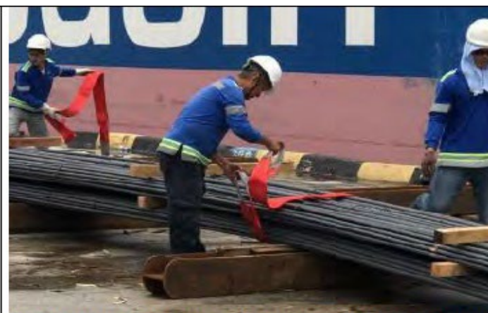
Pre-slugging of two tiers of rebars in preparation for loading.
