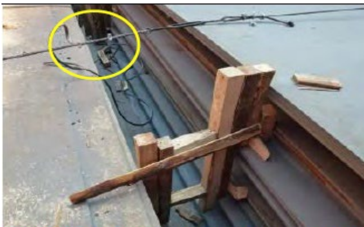
Correct use of dunnage. The dunnage is additionally secured horizontally. Incorrect use of bulldog grips on the left wire.
