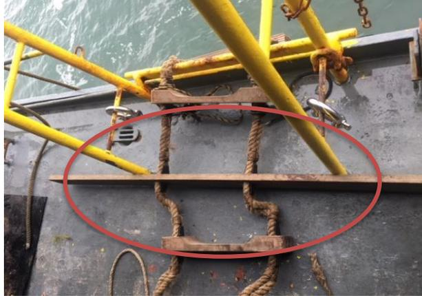
This example shows the completely unacceptable practice of bracing a spreader against the stanchion of the handrail.
