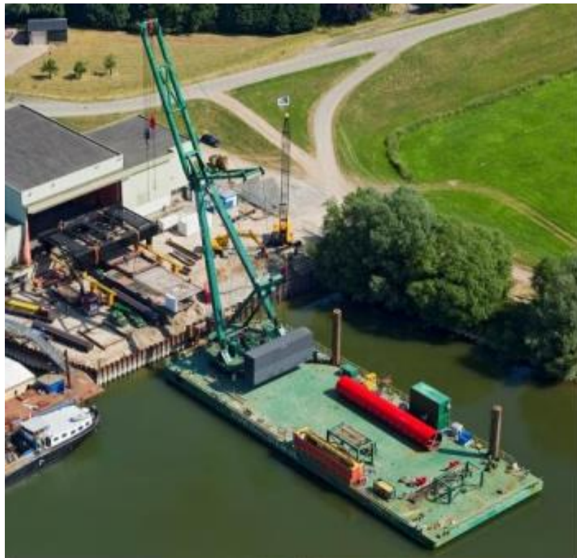
Skylift Crane Barge
