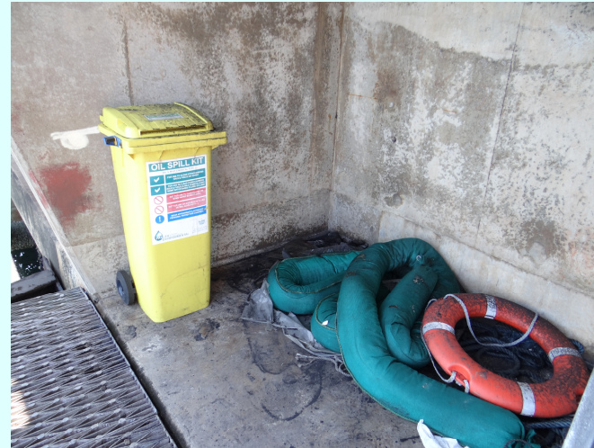
Photo Showing Oil Spill Response Kit Bins at Hunterston Jetty - Pilot Cutter Steps , August 2014
