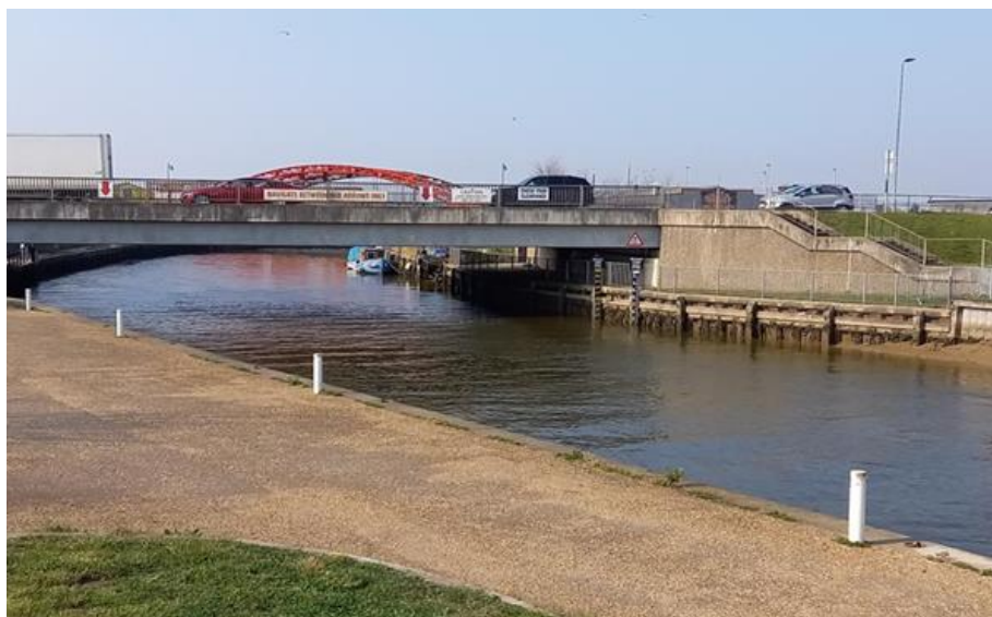
Acle Road Bridge viewed from N (upstream)
