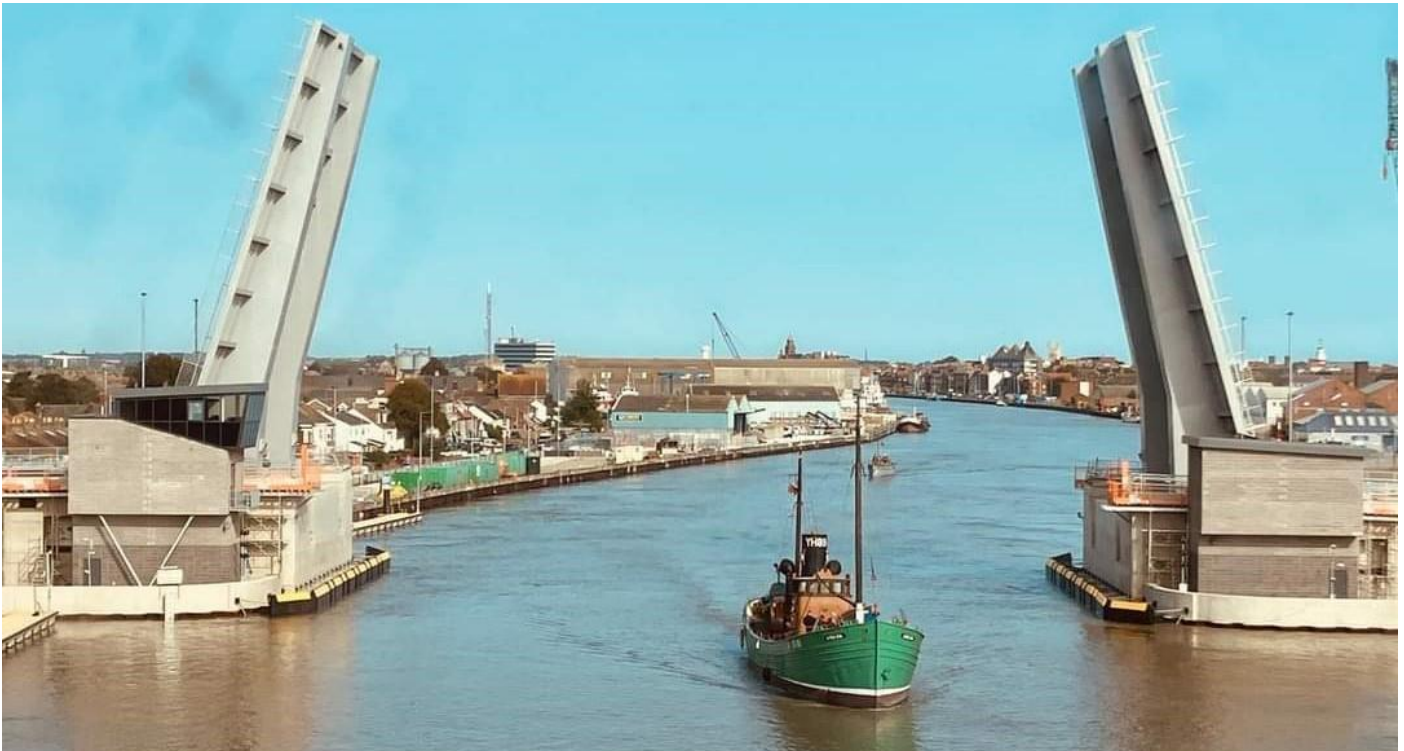
Herring Bridge viewed from S (seaward)
