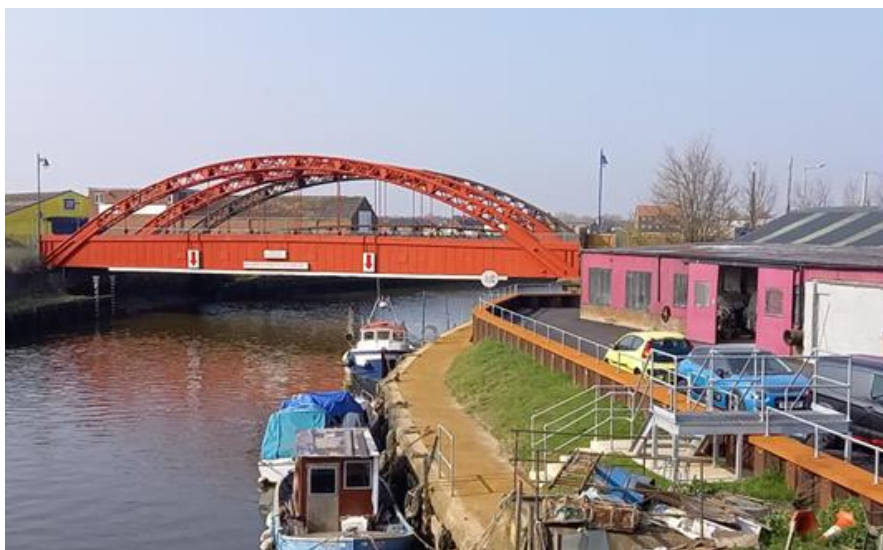
Vauxhall Bridge viewed from N (upstream)
