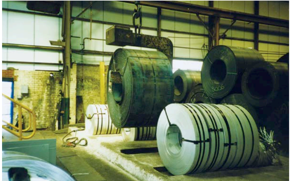
Photograph 15 Concrete coil wells for broad and narrow coils
