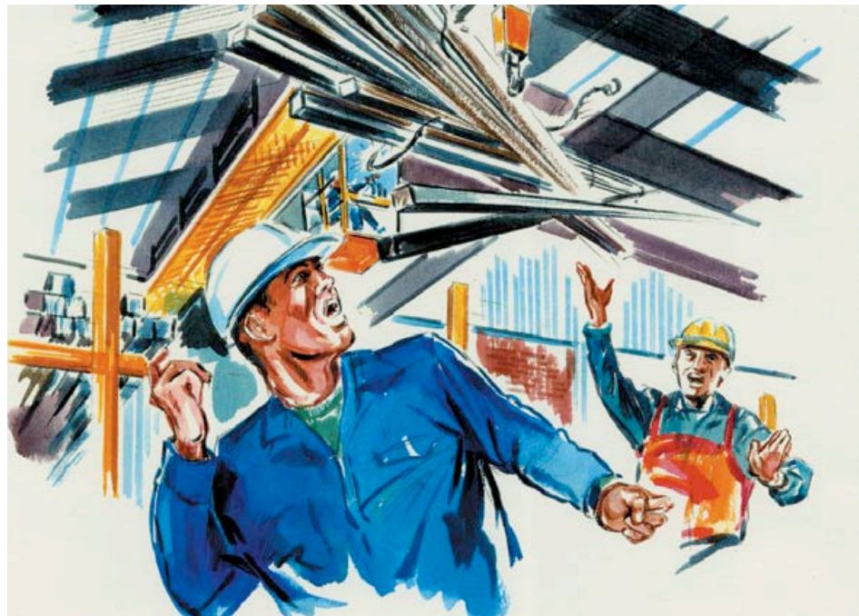
Figure 16 Collapse of bundle being lifted by banding.
