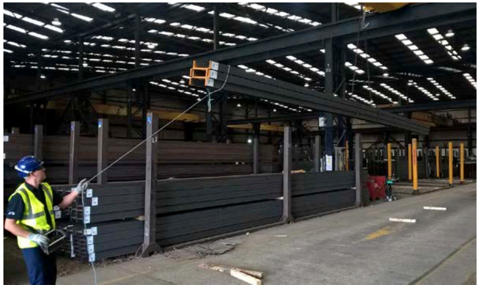
Photograph 28 Bundle of long product being lifted by an overhead crane. The operator is in a safe position, using a tag line to manoeuvre it into position
