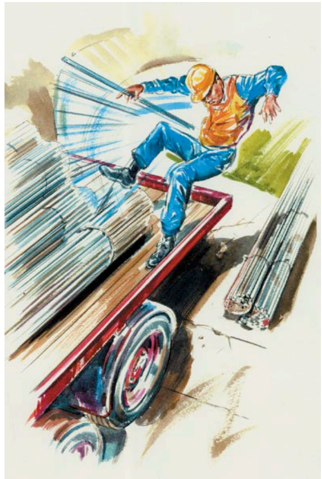
Figure 20 Unsafe system of work. Fall from lorry during barring-off of bundled stock
