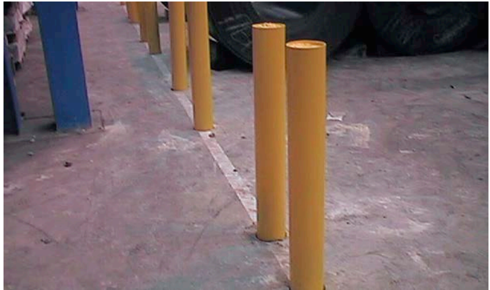
Photograph 12 Solid uprights for containing stock, (eg chocked broad coils) within storage areas
